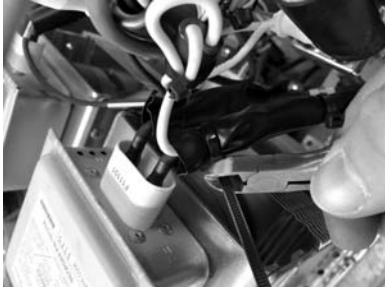
Figure 15 Securing and Trimming Cable Ties
