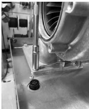
Figure 4 Removing Bolts and Washers
