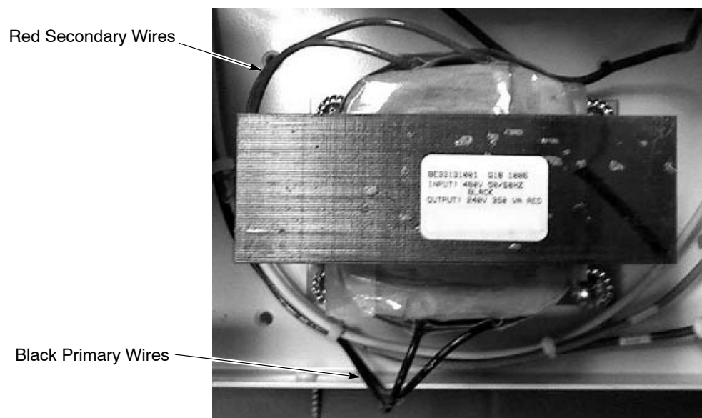
Figure 4 Cutting Old Transformer Wires
