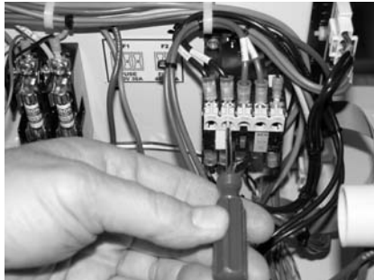
Loosen Terminal Screws
