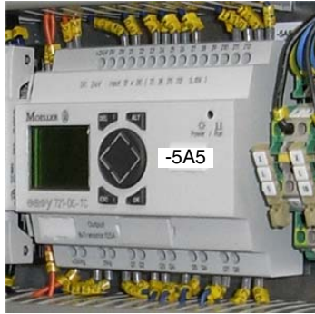
Fig. 3-9 Control relay
