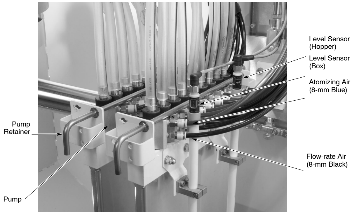
Figure 3-4 Pump, Air Tubing, and Powder Feed Hose Installation
