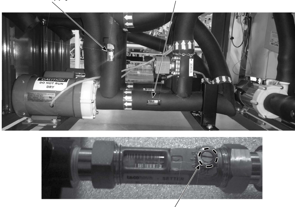
Chilled Water Supply Flowsetter Process Return Water Flowsetter
