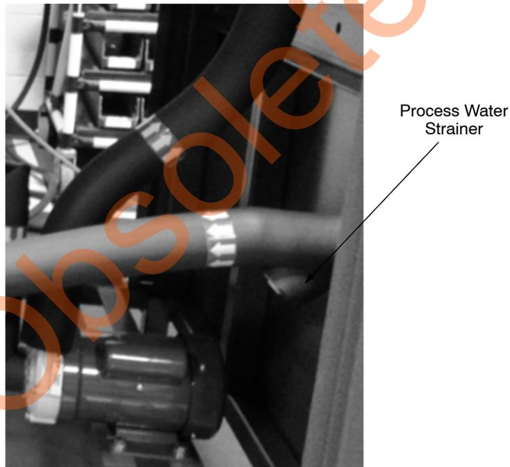
Figure 9 Process Water Strainer
