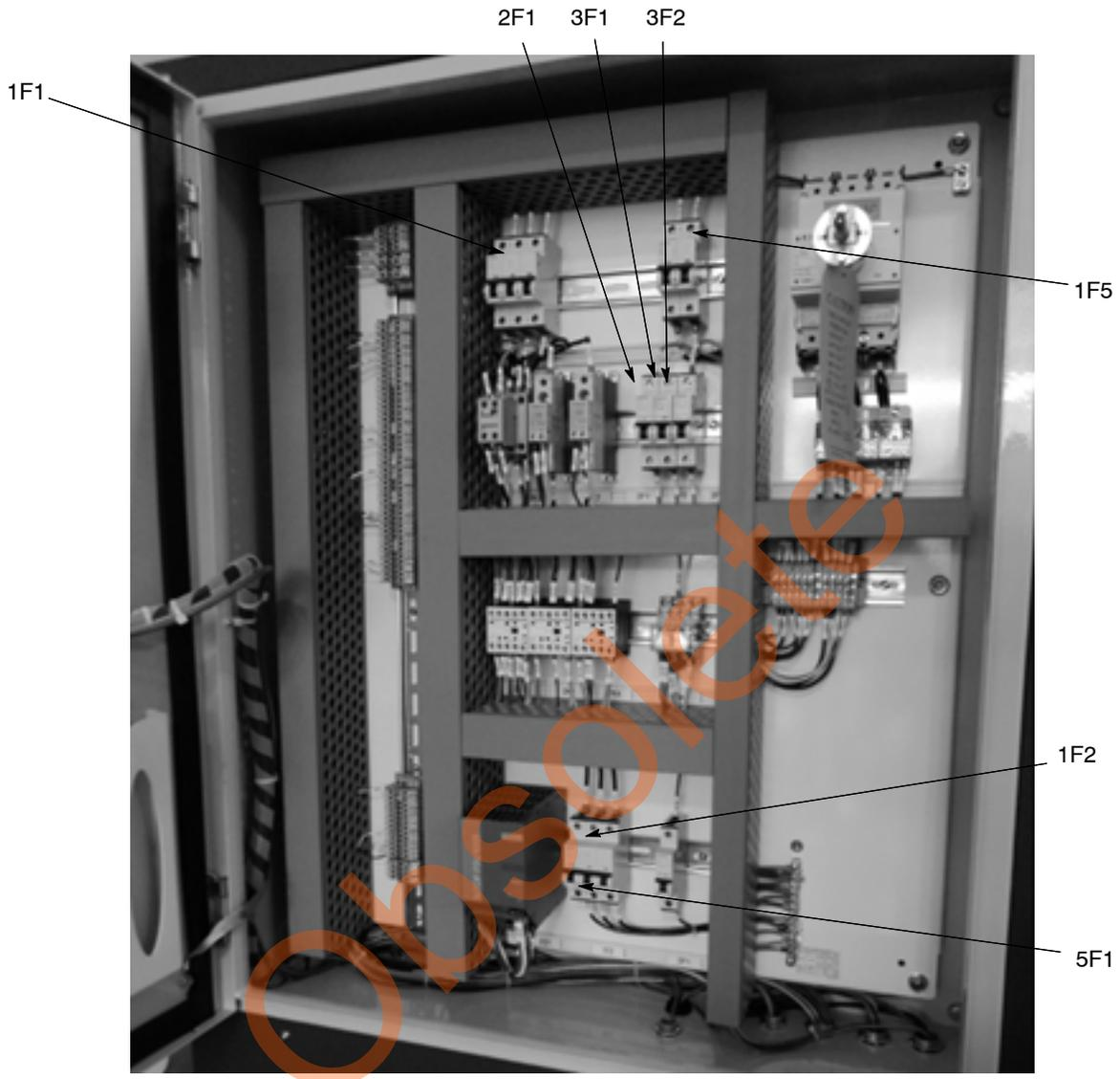
Figure 4 Control Panel Interior Fuses, Disconnects, and Controls
