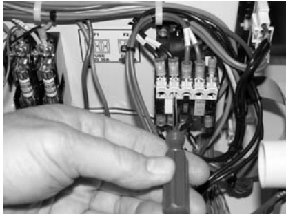
Loosen Terminal Screws
