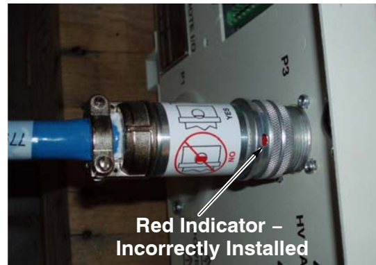
Figure 3-5 Unicable connector partially installed
